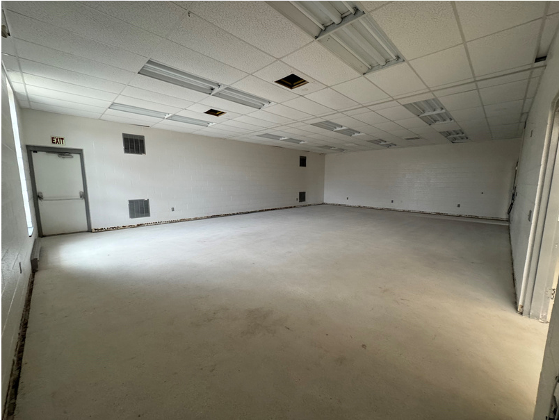
Conference room, post-asbestos remediation.
