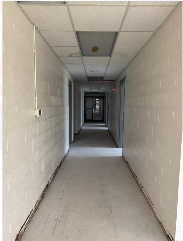
Hallway to PD, post-asbestos remediation.
