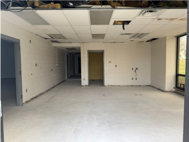
Front entrance, post-asbestos remediation.
