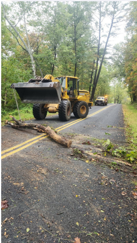
Maintenance to the rescue!
